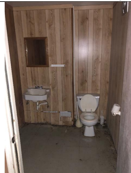
400 Mudd Ave - Bathroom
