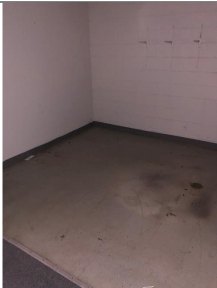
400 Mudd Ave – North Storage
